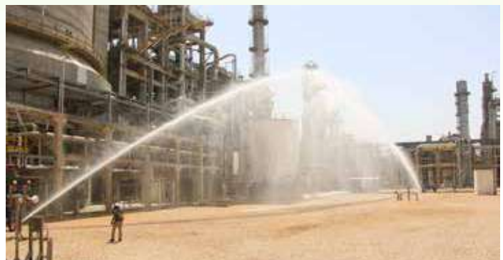
Fire water curtain formation by emergency team
